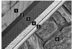
[1] Sheathing, [2] SM-BT, [3] Galvanized [1] Sheathing, [2] 10mm P.T. wood strapping, [1] Sheathing, [2] SM-BT, [3] Drainage mat, metal lath, [4] Mortar/scratch coat, [5] Mortar setting bed, [6] NTSV
