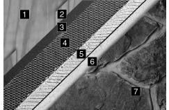
[3] SM-BT, [4] Galvanized metal lath, [5] [4] Galvanized metal lath, [5] Mortar/scratch Mortar/scratch coat, [6] Mortar setting bed, coat, [6] Mortar setting bed, [7] NTSV [7] NTSV
